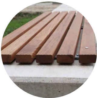
TIMBER HARDWOOD SLATS Timber slats fixed to stone or concrete
