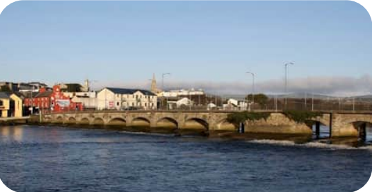
The Nineteen Arches Bridge
